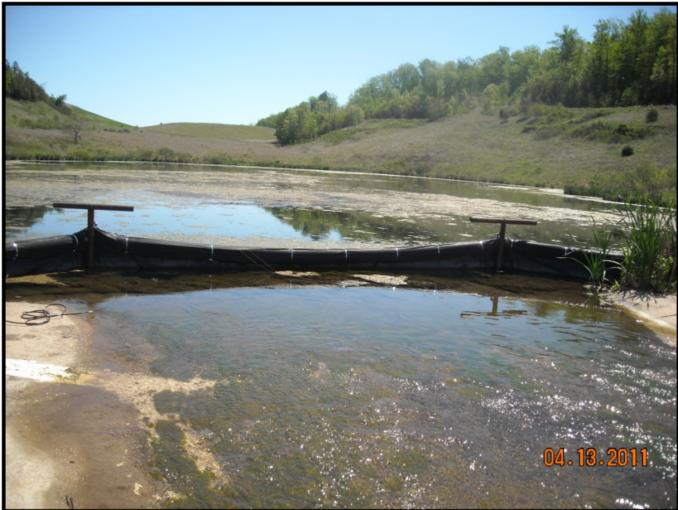
Photo B.243 – Treatment Pond Outfall DRMW-3 – Looking upstream – April 13, 2011
