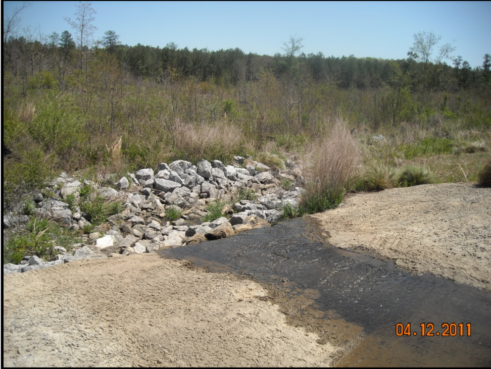
Photo B.260 – Treatment Pond Outfall DRMW-12 – Looking upstream – April 12, 2011
