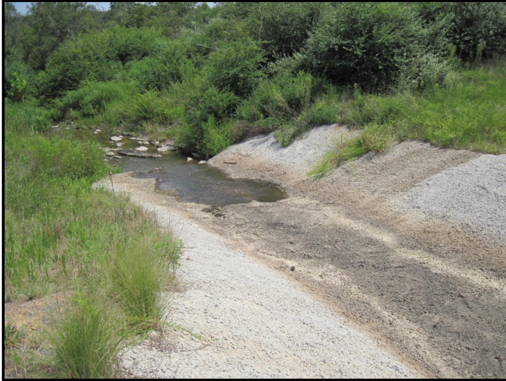
Photo B.224 – Treatment Pond Outfall BMWW-36 – Looking downstream – August 22, 2011
