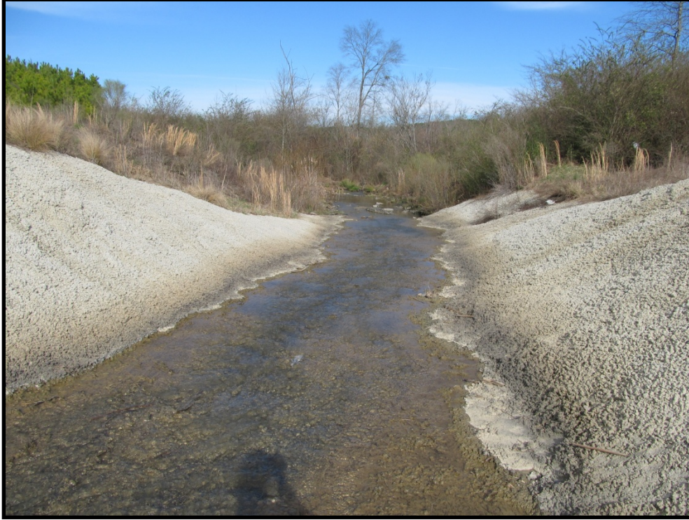
Photo B.228 – Treatment Pond Outfall BMWW-36 – Looking downstream – February 6, 2013
