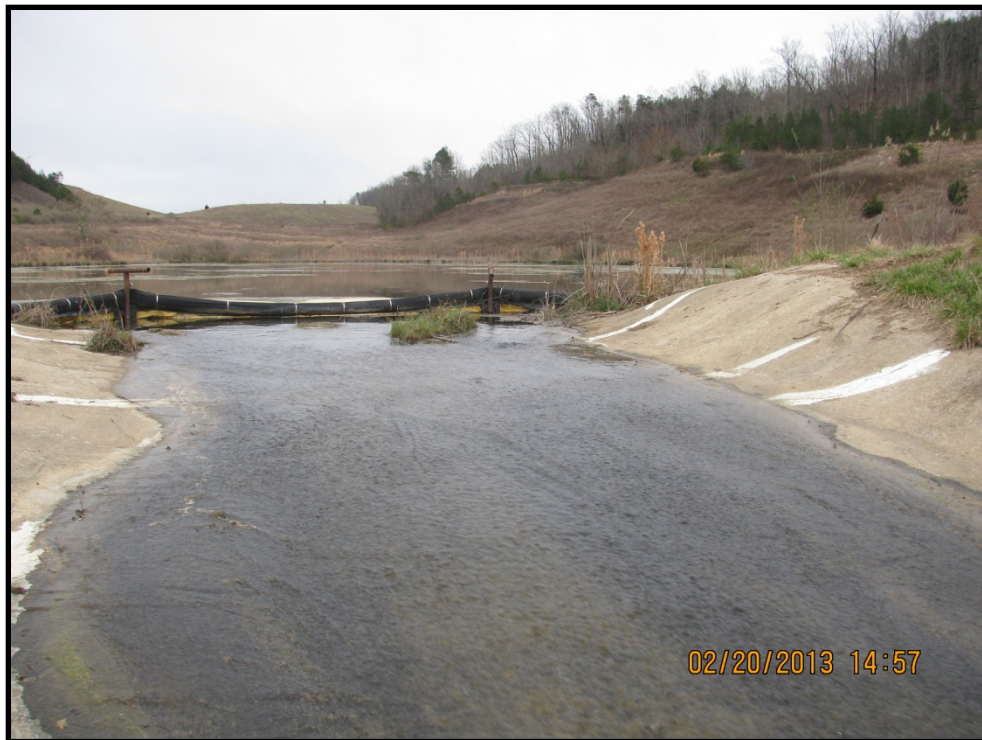
Photo B.255 – Treatment Pond Outfall DRMW-3 – Looking upstream – February 20, 2013
