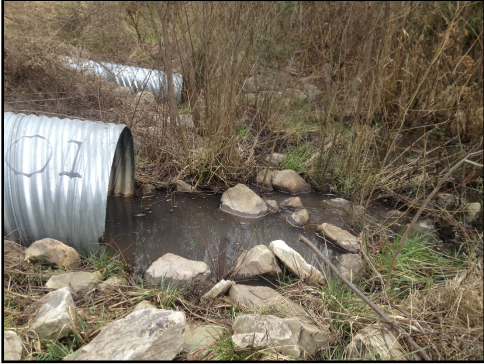
Photo B.280 – Treatment Pond Outfall WIMJ-1 – Discharge from pond – January 23, 2013
