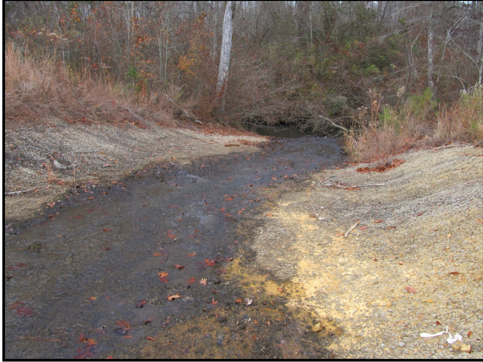
Photo B.206 – Treatment Pond Outfall BMWW-21 – Looking downstream – December 4, 2012
