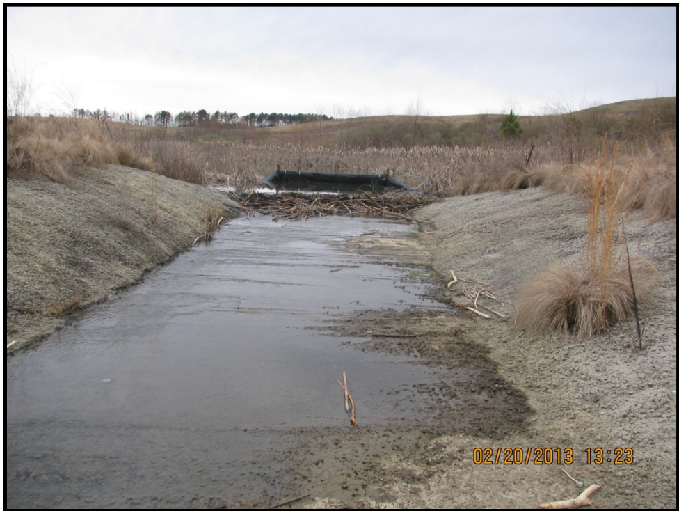
Photo B.271 – Treatment Pond Outfall DRMW-12 – Looking upstream – February 20, 2013 (Note - Beaver dam across weir)
