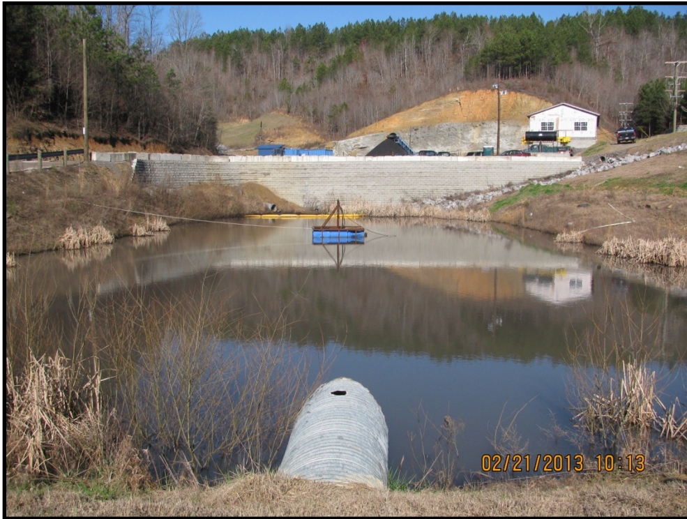
Photo B.281 – Treatment Pond Outfall WIMJ-1 – Looking upstream – February 21, 2013
