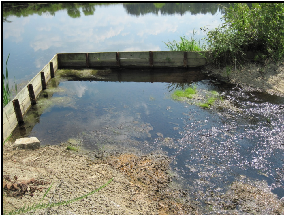
Photo B.203 – Treatment Pond Outfall BMWW-21 – Looking upstream – August 22, 2011
