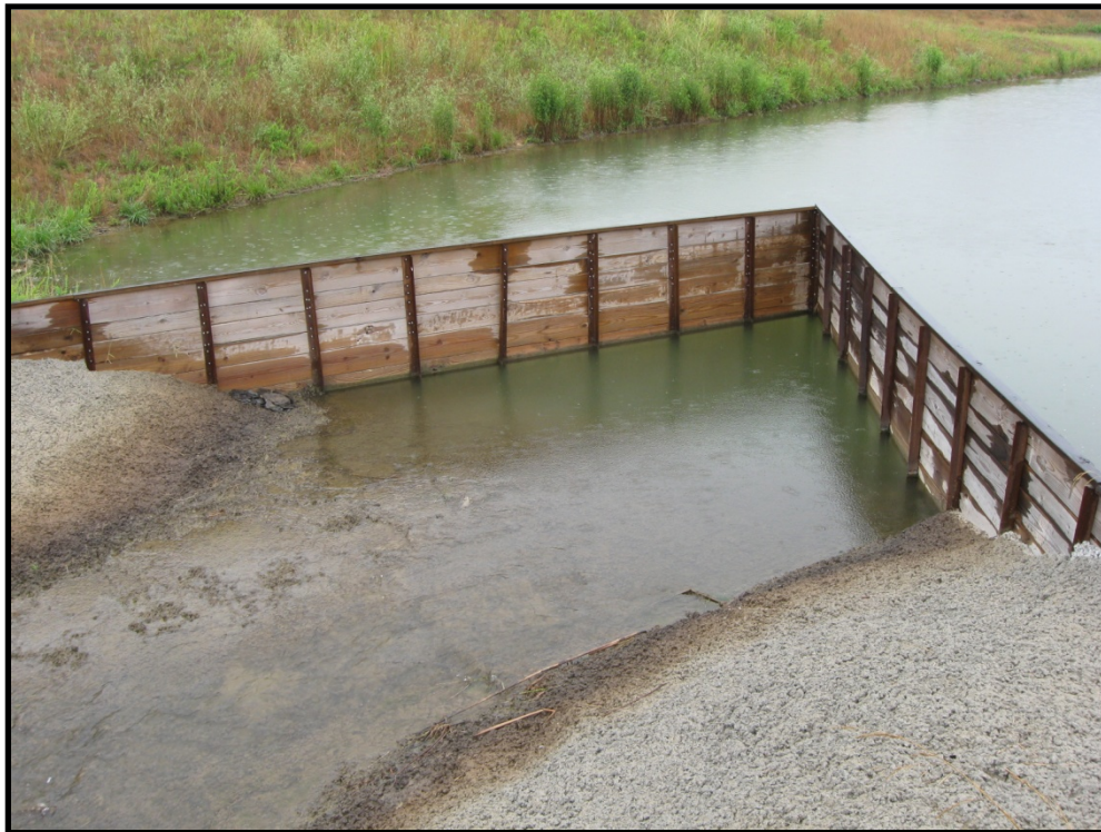
Photo B.219 – Treatment Pond Outfall BMWW-36 – Looking upstream – June 28, 2011
