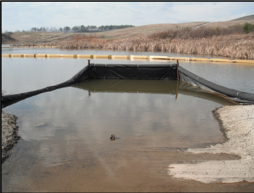
Photo B.257 – Treatment Pond Outfall DRMW-12 – Looking upstream – February 24, 2011
