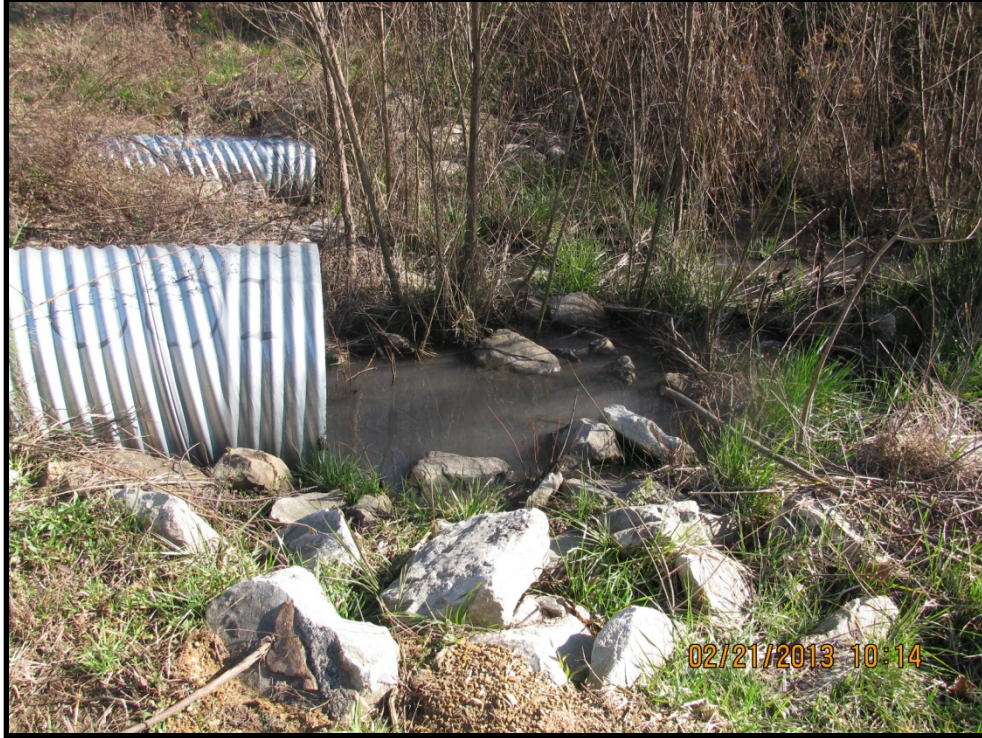
Photo B.282 – Treatment Pond Outfall WIMJ-1 – Discharge from pond – February 21, 2013
