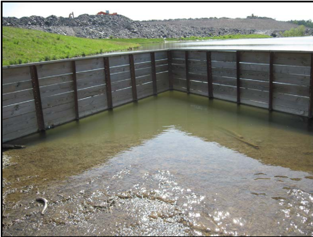
Photo B.215 – Treatment Pond Outfall BMWW-36 – Looking upstream – April 14, 2011
