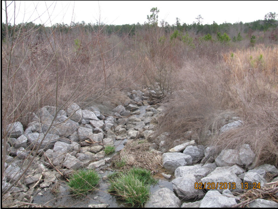
Photo B.272 – Treatment Pond Outfall DRMW-12 – Looking downstream – February 20, 2013
