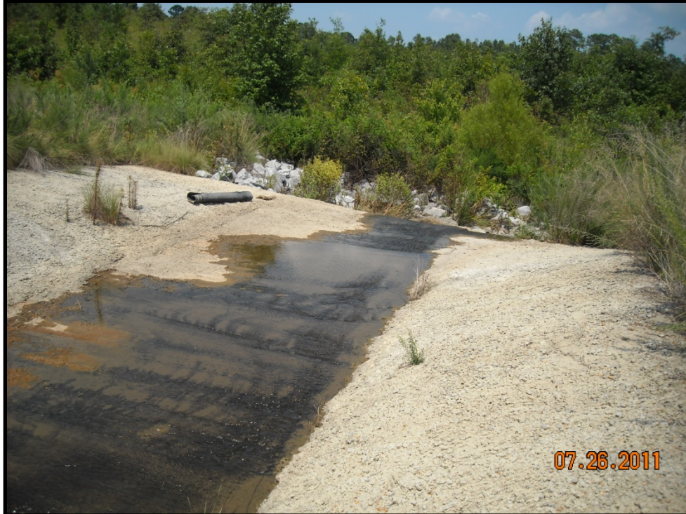
Photo B.264 – Treatment Pond Outfall DRMW-12 – Looking downstream – July 26, 2011
