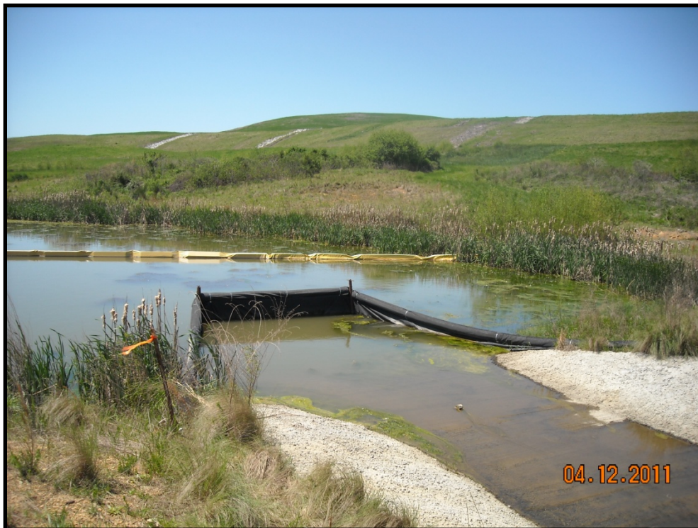
Photo B.259 – Treatment Pond Outfall DRMW-12 – Looking upstream – April 12, 2011
