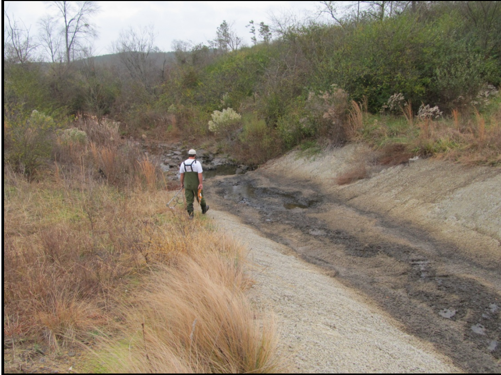
Photo B.226 – Treatment Pond Outfall BMWW-36 – Looking downstream – December 4, 2012
