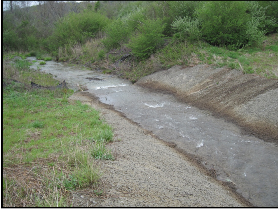
Photo B.214 – Treatment Pond Outfall BMWW-36 – Looking downstream – March 30, 2011
