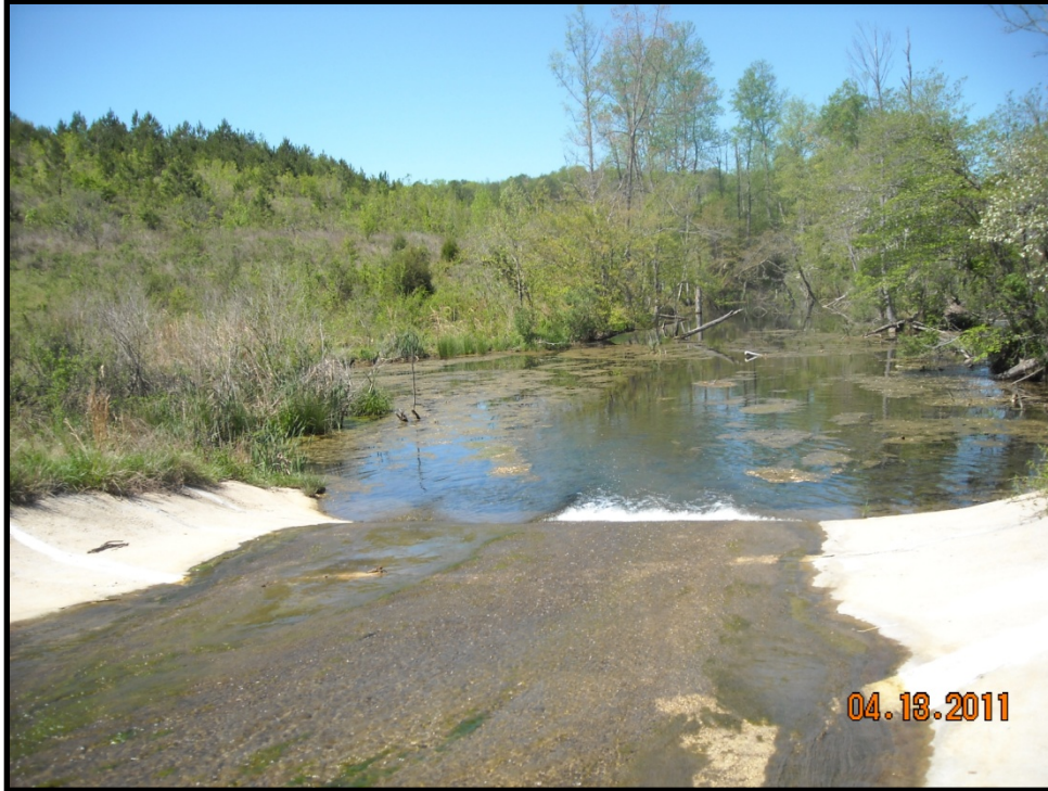
Photo B.244 – Treatment Pond Outfall DRMW-3 – Looking downstream – April 13, 2011
