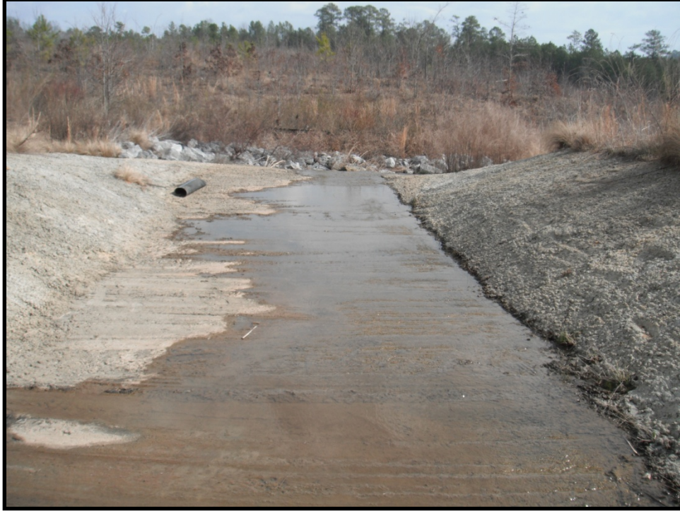
Photo B.258 – Treatment Pond Outfall DRMW-12 – Looking downstream – February 24, 2011
