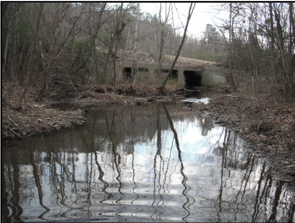
Photo B.130 – Coal Creek (CLCJ-3) – Looking downstream – February 25, 2011
