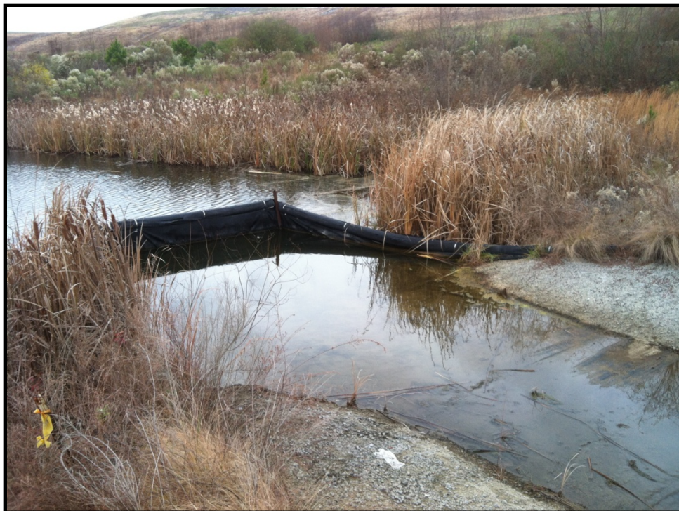
Photo B.267 – Treatment Pond Outfall DRMW-12 – Looking upstream – December 4, 2012
