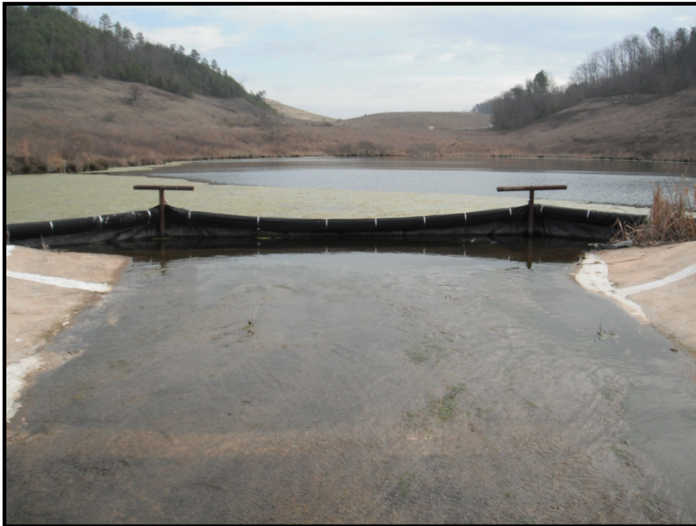
Photo B.241 – Treatment Pond Outfall DRMW-3 – Looking upstream – February 24, 2011
