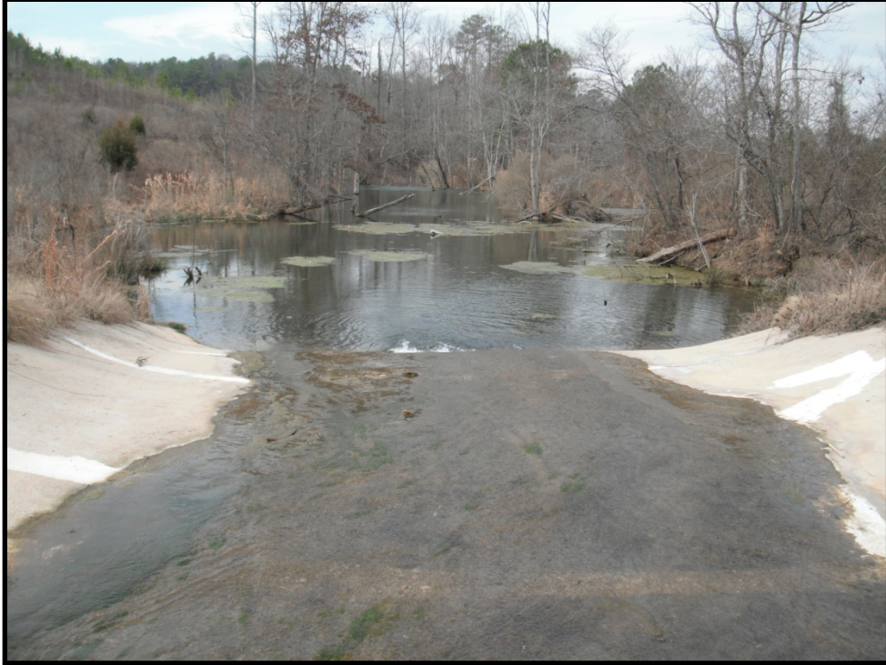
Photo B.242 – Treatment Pond Outfall DRMW-3 – Looking downstream – February 24, 2011
