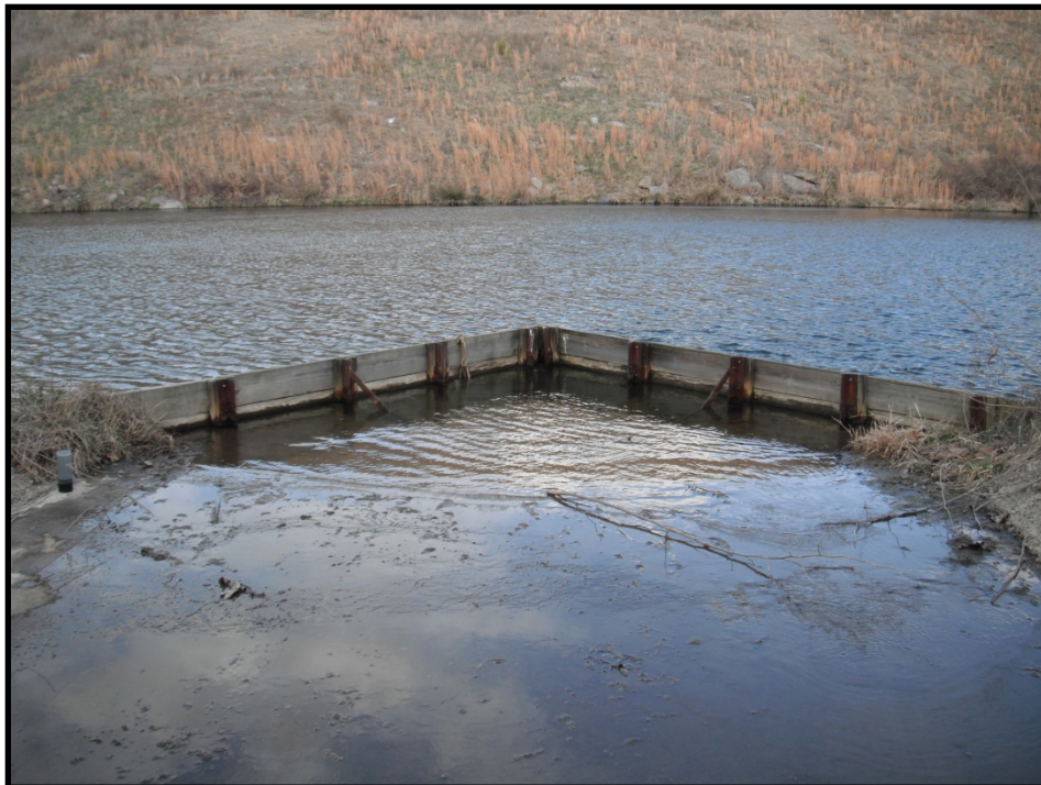
Photo B.229 – Treatment Pond Outfall CHMJ-47 – Looking upstream – February 24, 2011
