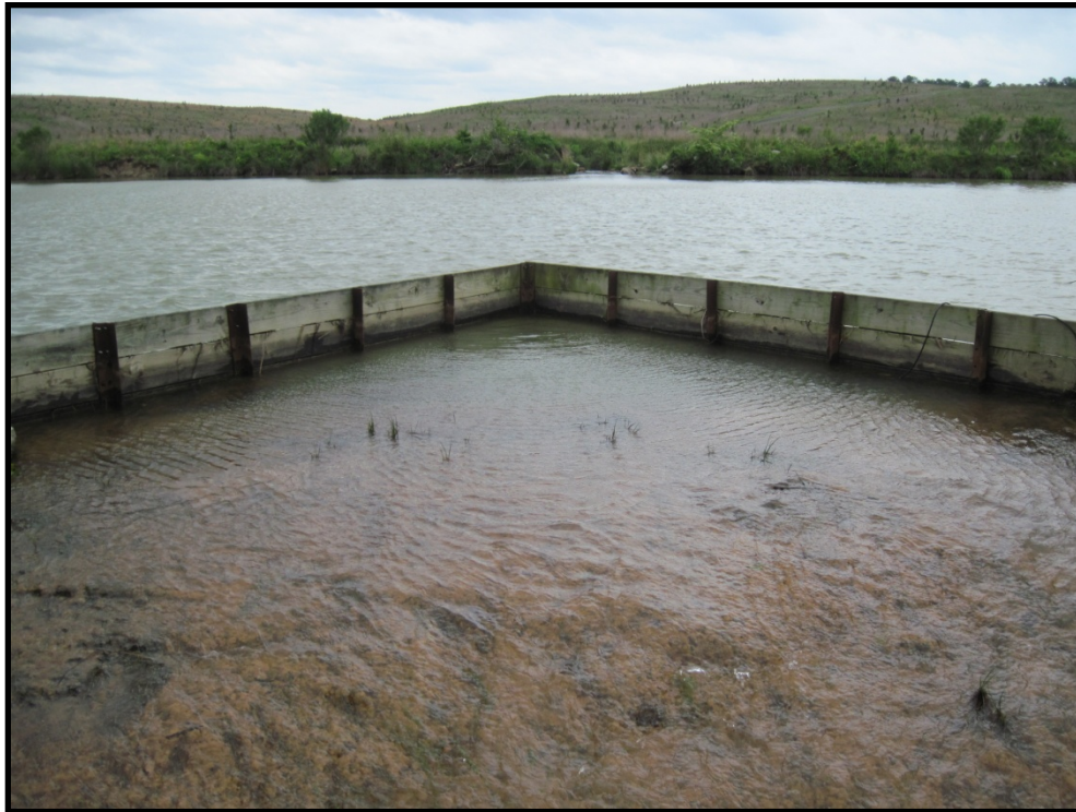
Photo B.195 – Treatment Pond Outfall BMWW-21 – Looking upstream – April 27, 2011
