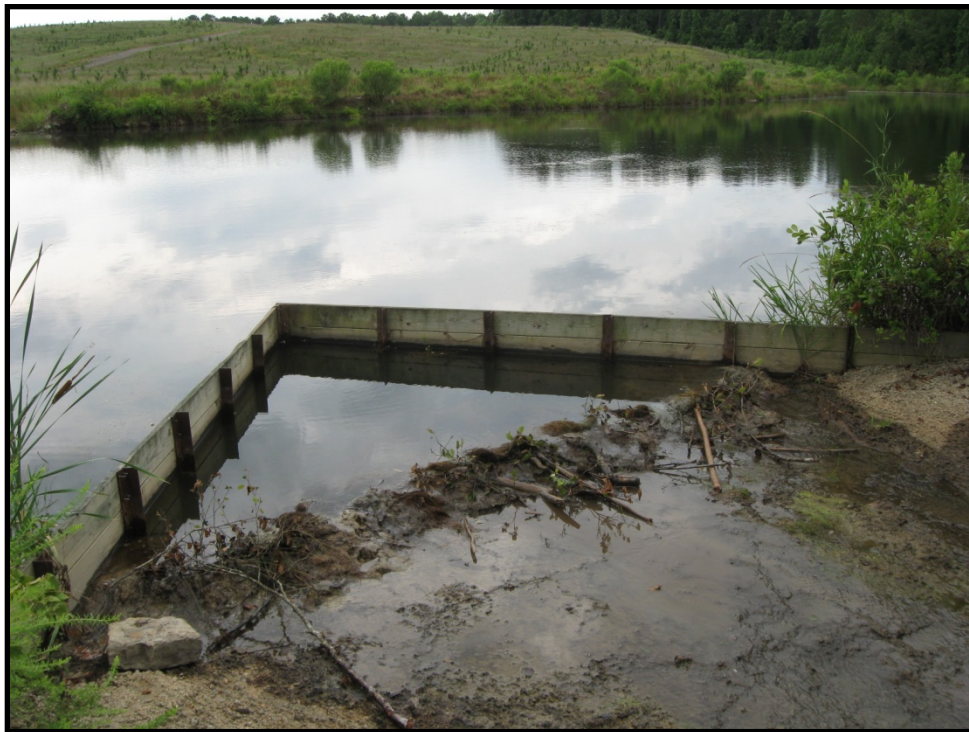
Photo B.199 – Treatment Pond Outfall BMWW-21 – Looking upstream – June 28, 2011
