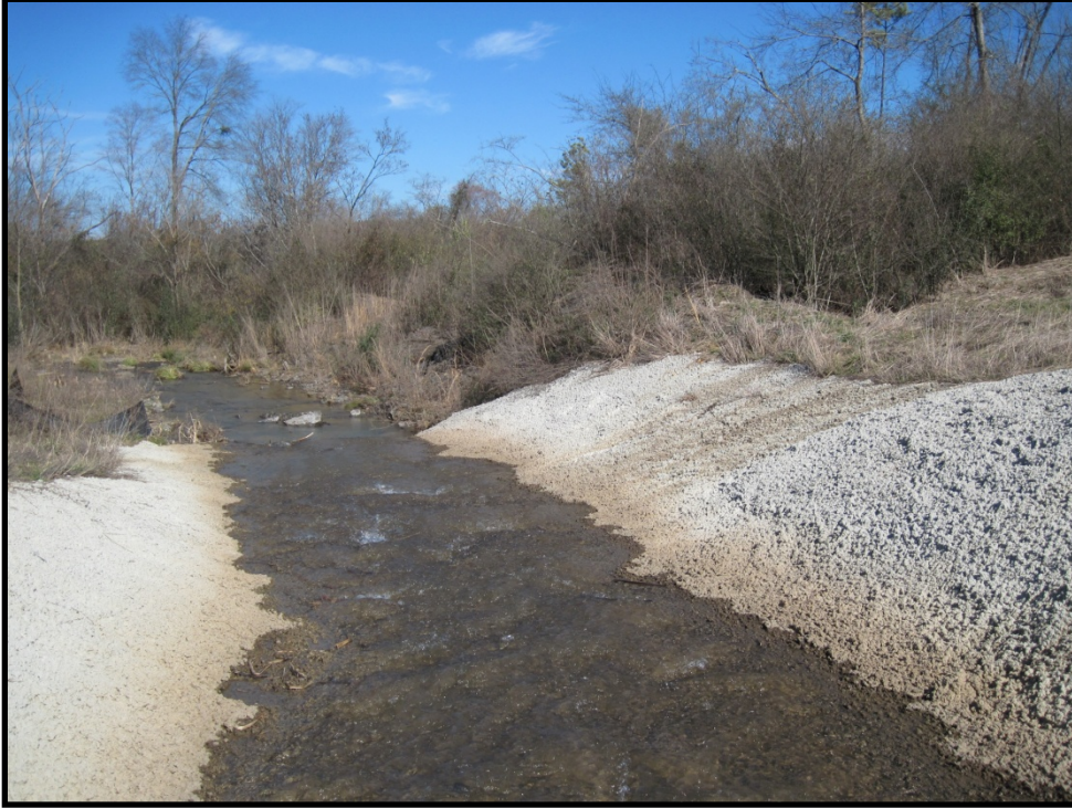
Photo B.212 – Treatment Pond Outfall BMWW-36 – Looking downstream – February 22, 2011
