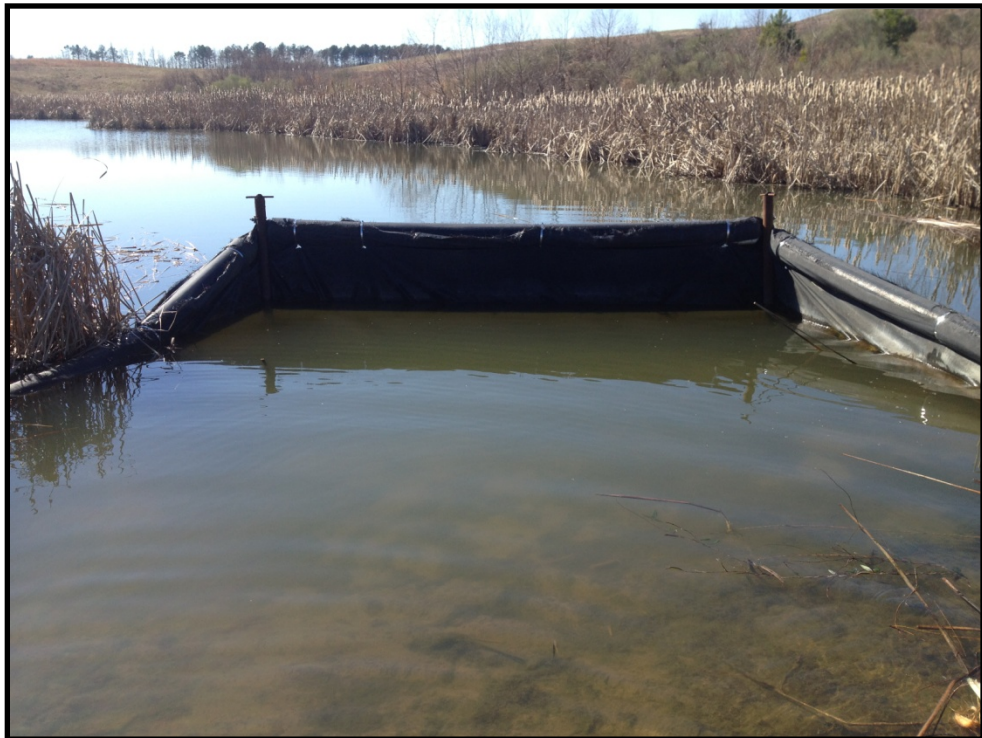
Photo B.269 – Treatment Pond Outfall DRMW-12 – Looking upstream – January 22, 2013
