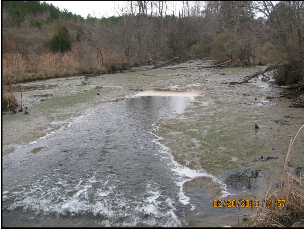
Photo B.256 – Treatment Pond Outfall DRMW-3 – Looking downstream – February 20, 2013
