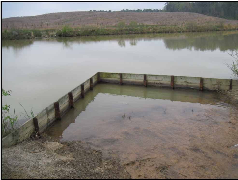
Photo B.193 – Treatment Pond Outfall BMWW-21 – Looking upstream – March 30, 2011
