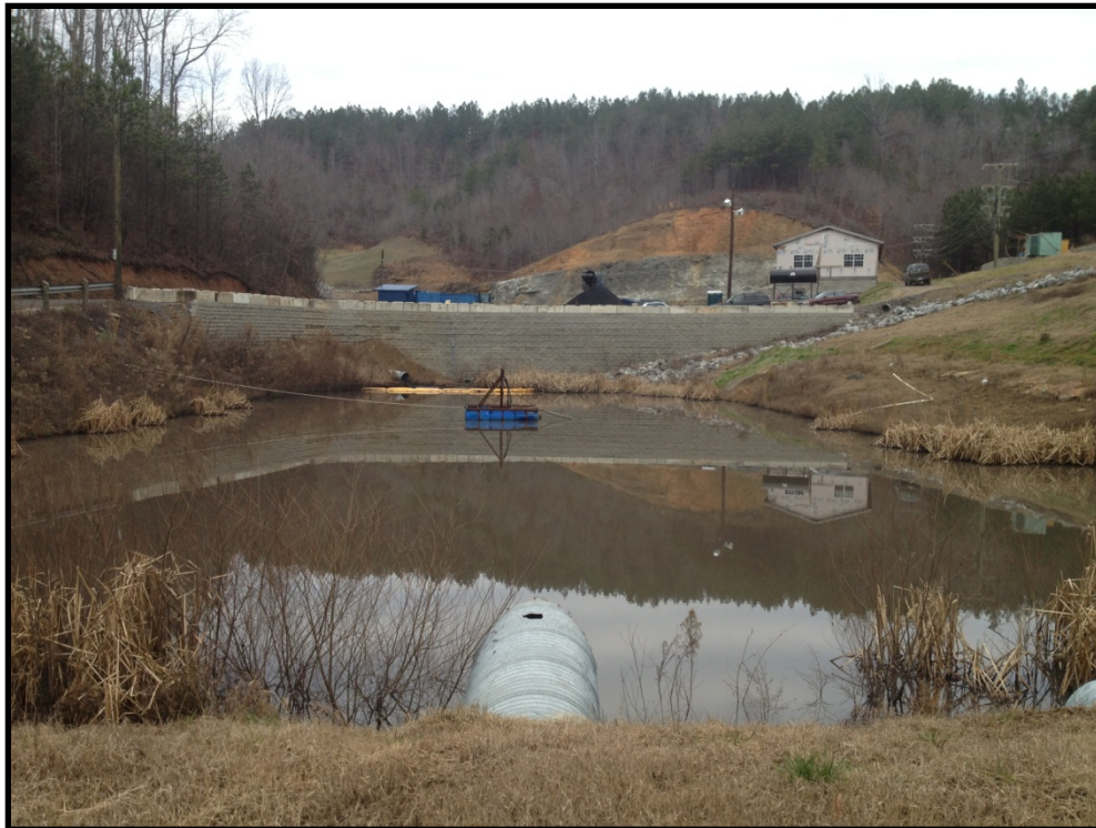
Photo B.279 – Treatment Pond Outfall WIMJ-1 – Looking upstream – January 23, 2013
