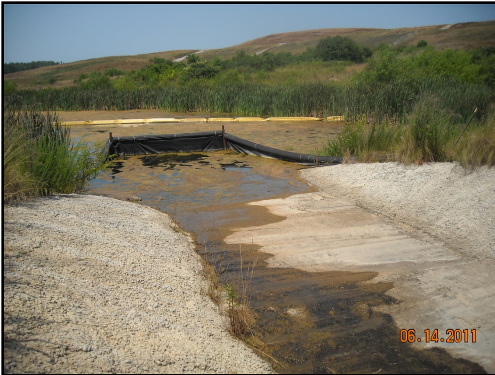
Photo B.261 – Treatment Pond Outfall DRMW-12 – Looking upstream – June 14, 2011
