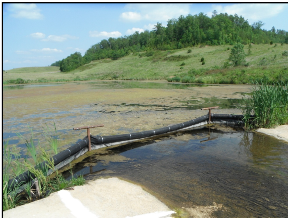
Photo B.245 – Treatment Pond Outfall DRMW-3 – Looking upstream – May 9, 2011
