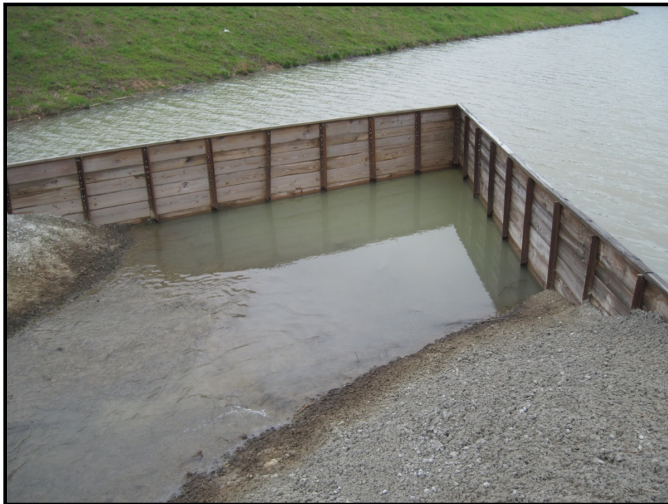
Photo B.213 – Treatment Pond Outfall BMWW-36 – Looking upstream – March 30, 2011
