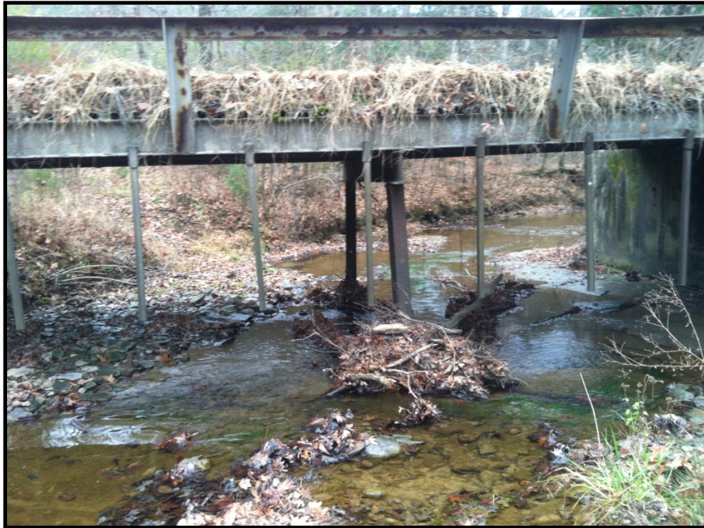
Photo B.52 – Burton Creek (BURW-1) – Looking downstream – December 4, 2012
