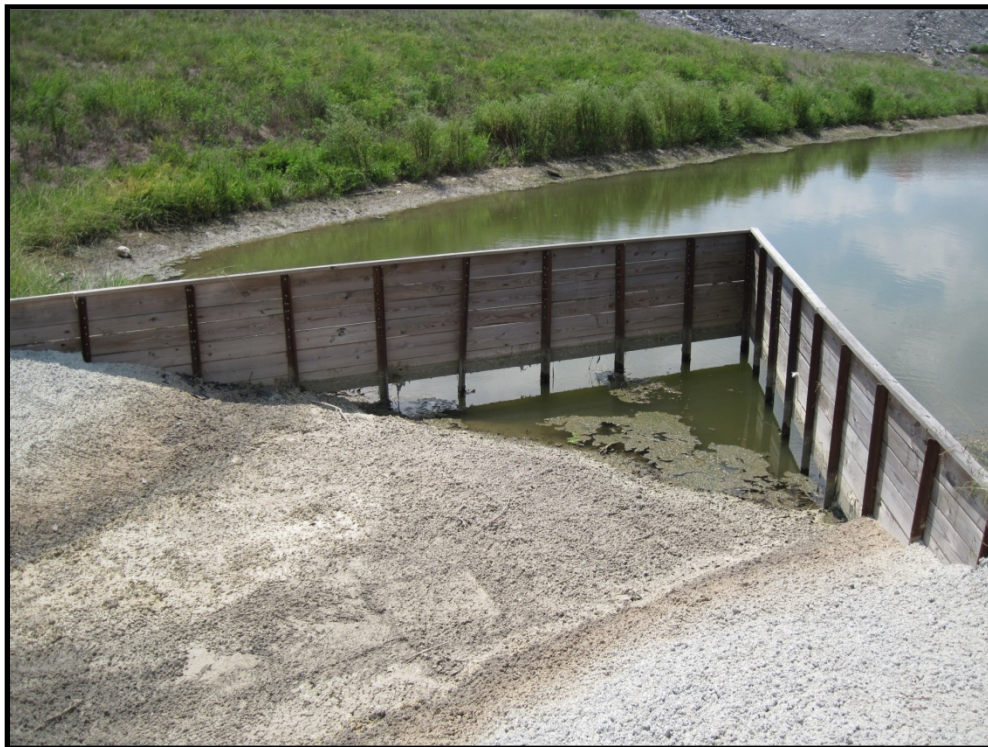
Photo B.223 – Treatment Pond Outfall BMWW-36 – Looking upstream – August 22, 2011
