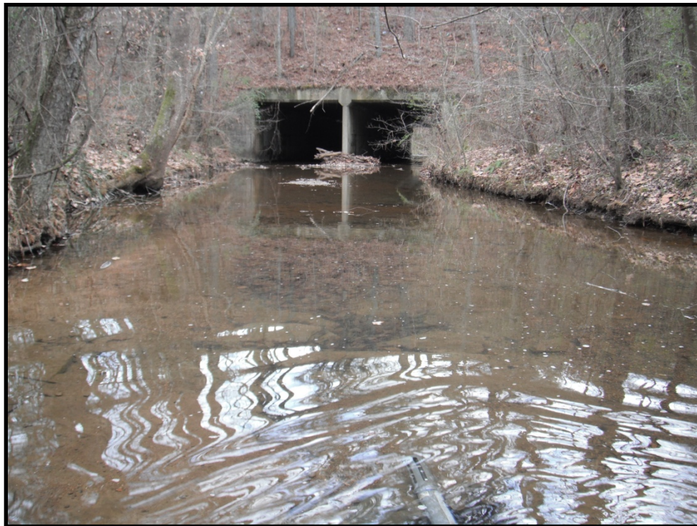
Photo B.120 – Coal Creek (CLCJ-1) – Looking downstream – February 25, 2011
