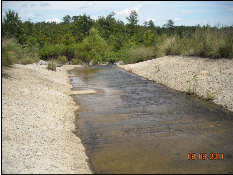
Photo B.266 – Treatment Pond Outfall DRMW-12 – Looking downstream – August 9, 2011
