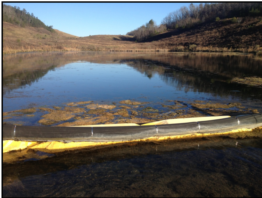
Photo B.251 – Treatment Pond Outfall DRMW-3 – Looking upstream – December 18, 2012
