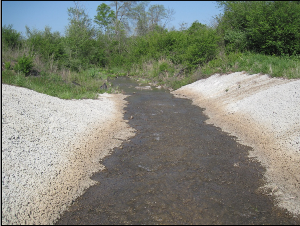
Photo B.216 – Treatment Pond Outfall BMWW-36 – Looking downstream – April 14, 2011
