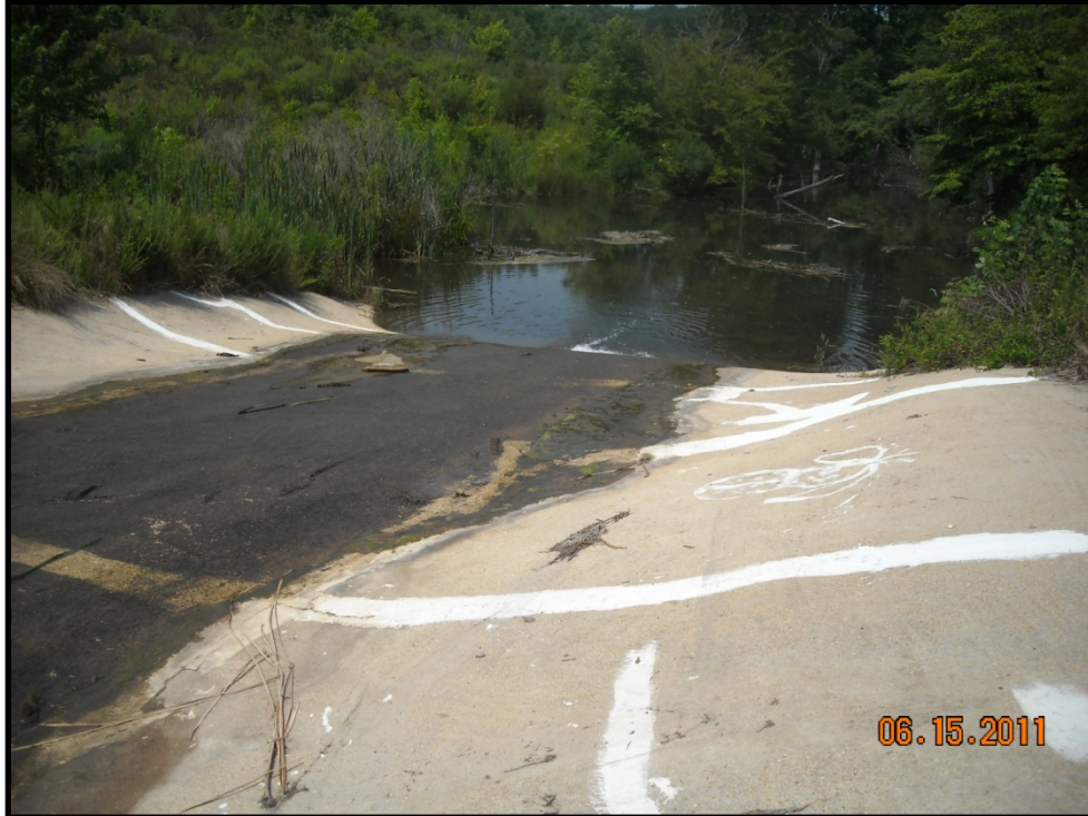
Photo B.248 – Treatment Pond Outfall DRMW-3 – Looking downstream – June 15, 2011
