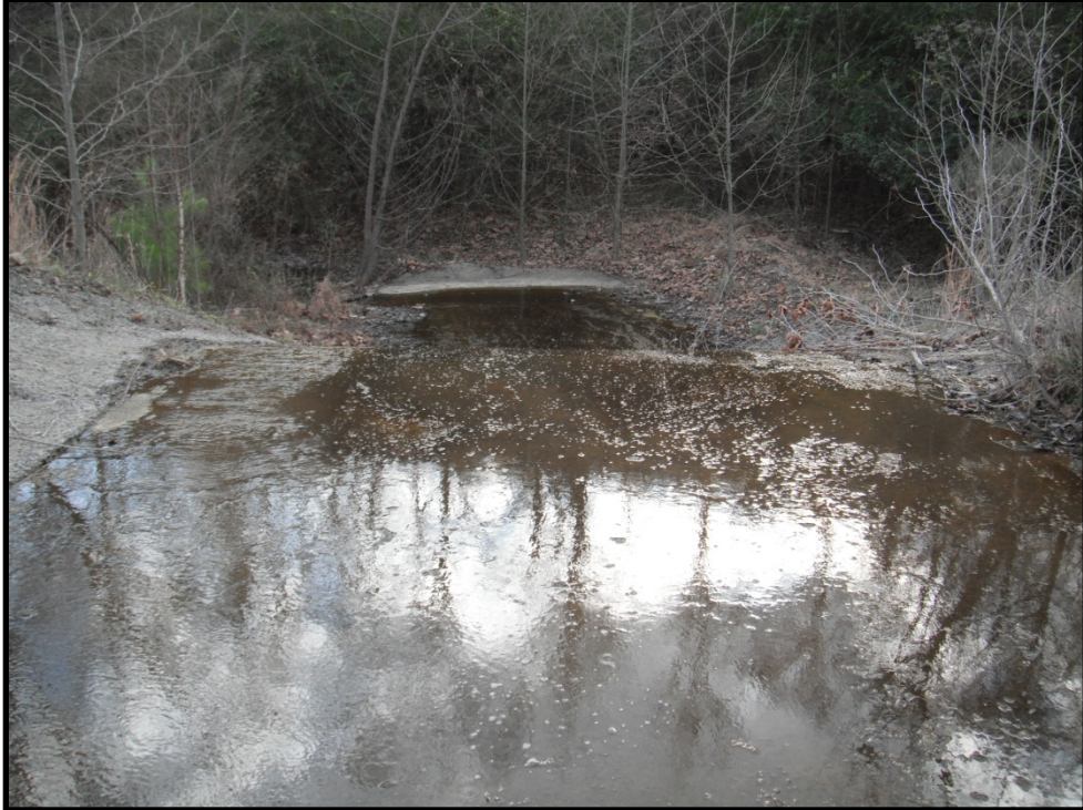
Photo B.230 – Treatment Pond Outfall CHMJ-47 – Looking downstream – February 24, 2011
