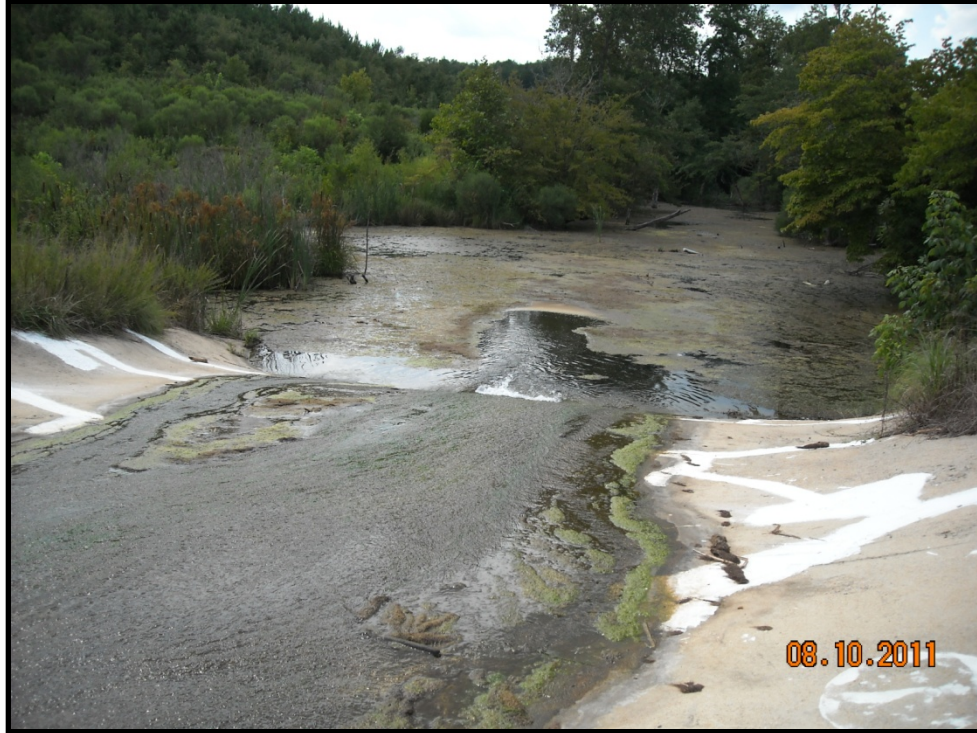
Photo B.250 – Treatment Pond Outfall DRMW-3 – Looking downstream – August 10, 2011
