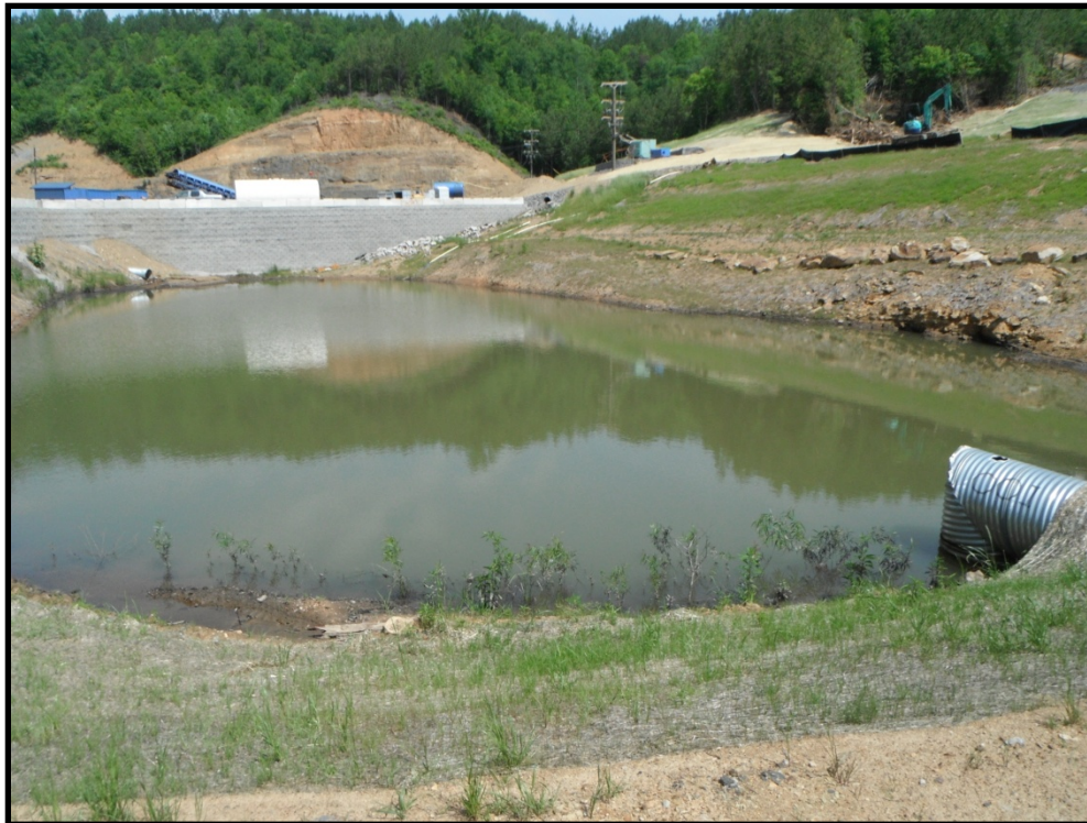
Photo B.275 – Treatment Pond Outfall WIMJ-1 – Looking upstream – May 9, 2011
