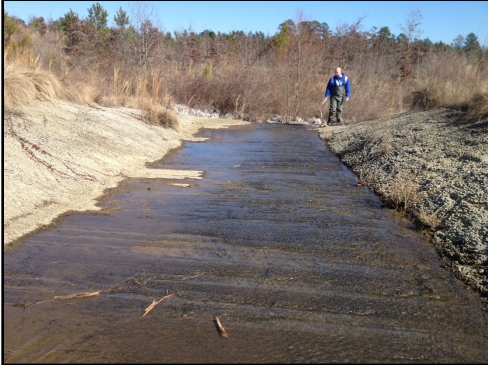
Photo B.270 – Treatment Pond Outfall DRMW-12 – Looking downstream – January 22, 2013
