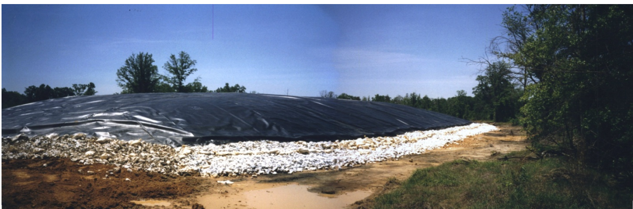
Brass foundry waste staged for removal
