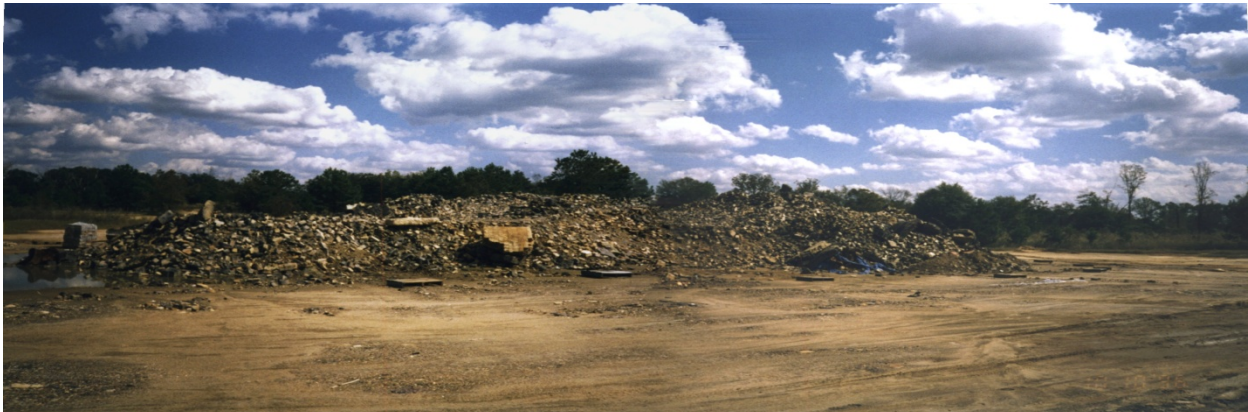
Foundry brick staged for removal
