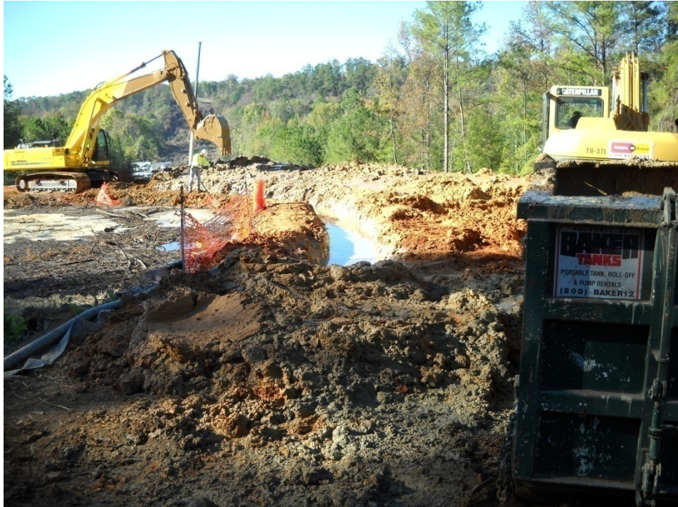
EPA constructing a slurry containment wall around the lagoons
