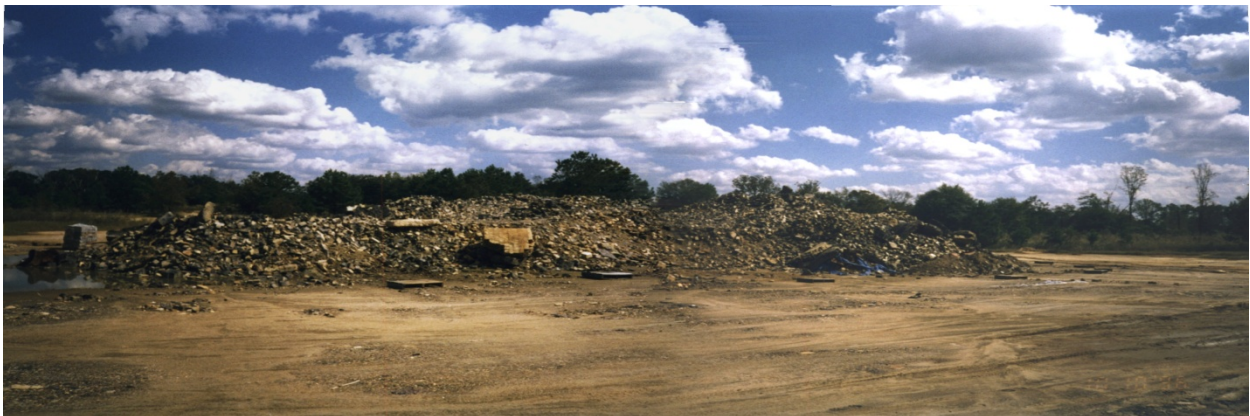
Foundry brick staged for removal
