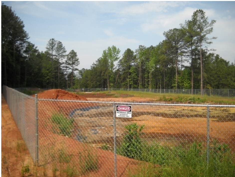
Completed slurry containment wall and enclosure
