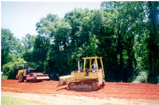
Backfilling of areas where contaminated soil was removed – Phillies Cigar, Dallas County
