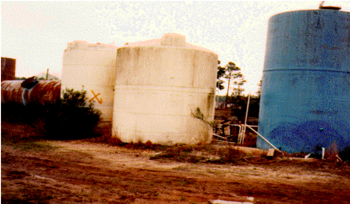
Caren Inc., tanks, Gulf Shores, Baldwin County, Alabama
