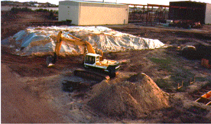
Excavation at the Alabama Shipyards
