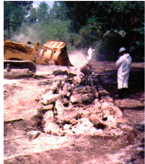
Excavation and destruction of dip vats at Cahaba Wood Preserving
