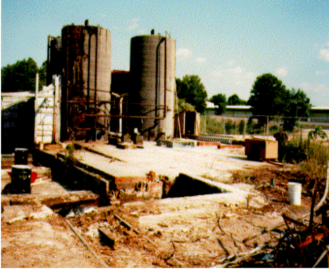
Fulco Lumber Company tanks prior to removal by EPA ERRB
