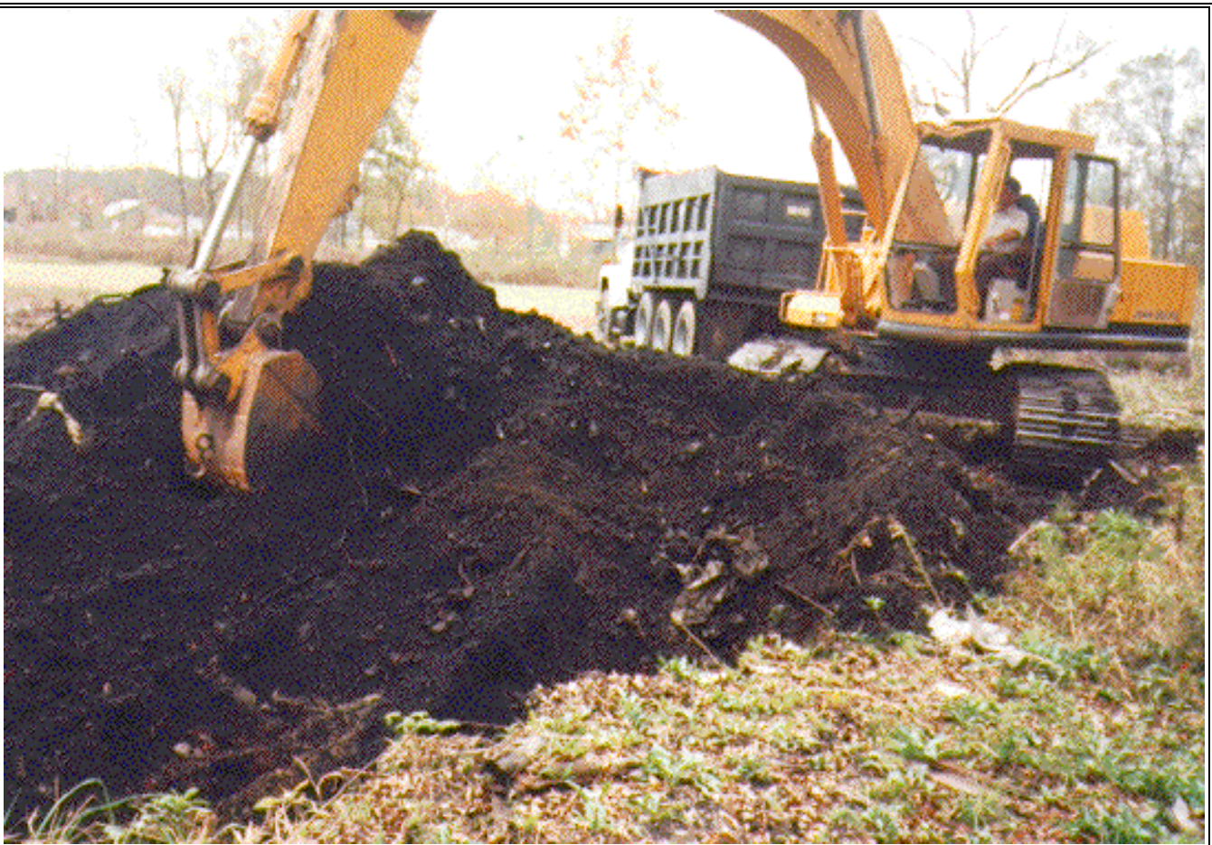
Scott Junkyard excavation, Brewton, Escambia County, Alabama
