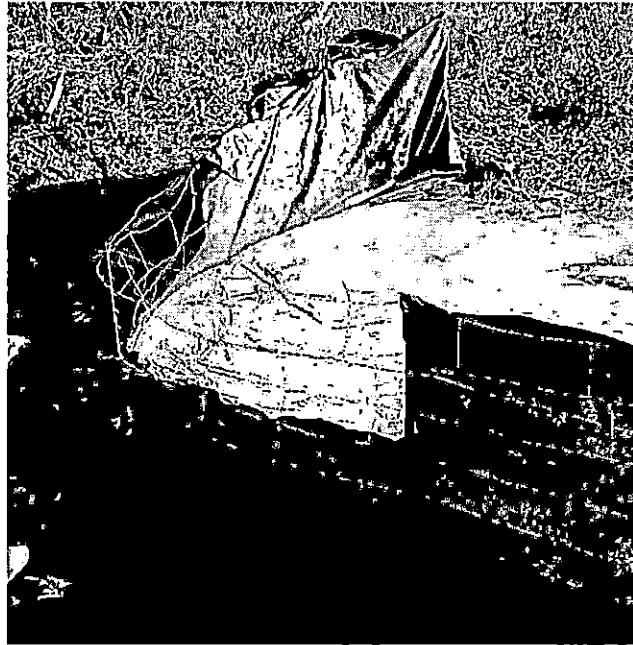
Figure CD-7 Silt Fence Check Dam (Photo courtesy of Auburn University SWRC)
