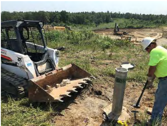
Photo #23 Removing concrete pad, well bollards, well vault, etc.
