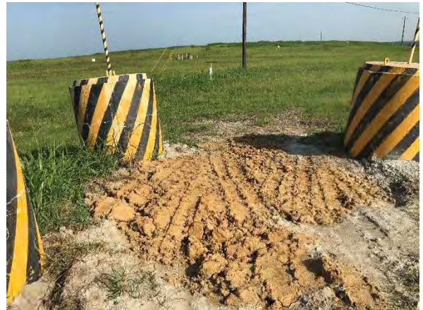
Photo #14 M-65 completed abandonment
