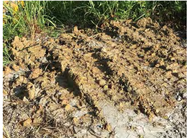
Photo #22 M-68 completed abandonment
