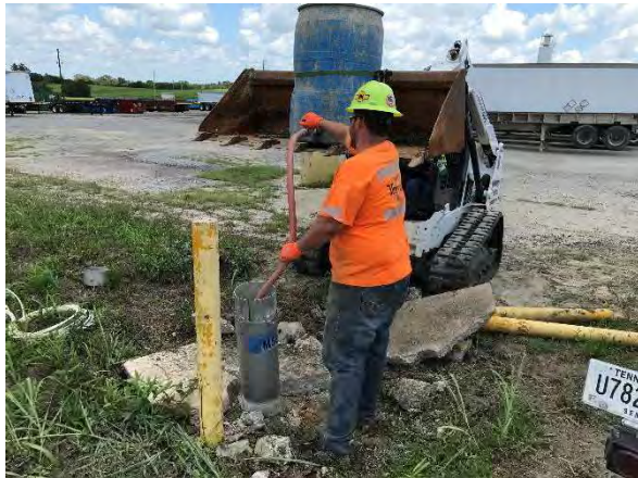
Photo #1 Method of grouting the M-series wells.
