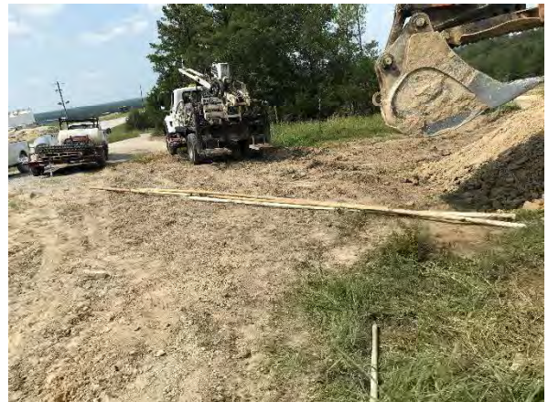
Photo #28 Located the break and removed the well casing.
