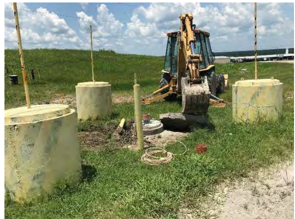
Photo #4 Method of removing concrete pad, well bollards, well vault, etc.
