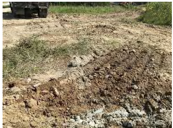
Photo #30 BG-1 completed abandonment.
