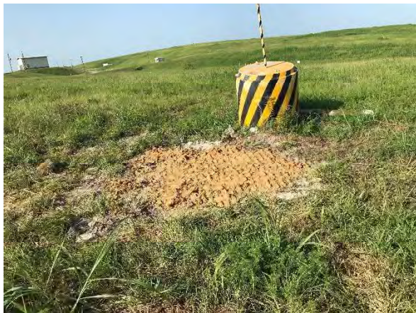
Photo #15 M-54 completed abandonment
