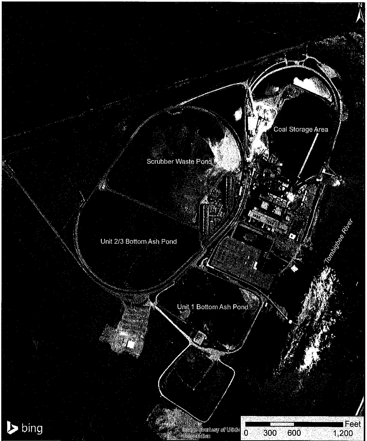
Figure 2 - Unit 1 Aerial Map of Impoundments Charles R. Lowman Power Plant PowerSouth Energy Cooperative Leroy, AL
