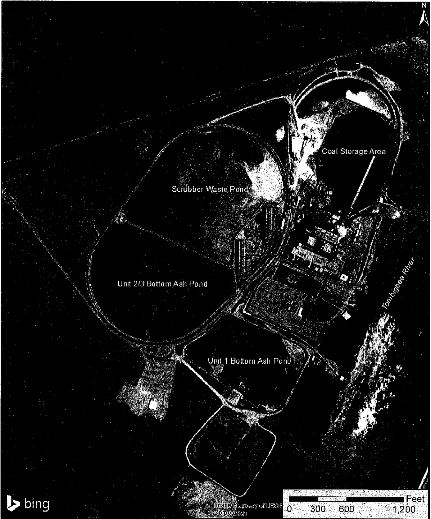
Figure 2 - Aerial Map of Impoundments Charles R. Lowman Power Plant PowerSouth Energy Cooperative Leroy, AL
