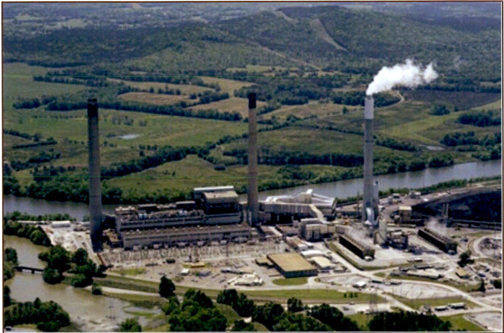
Figure 1: E.C. Gaston Steam Electric Generating Plant
