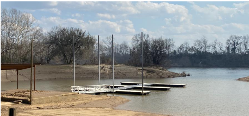
A new pier is under construction at the Selma Marina
